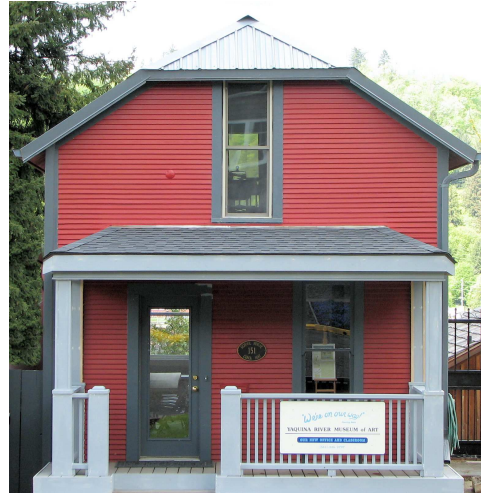
1887 School House Museum & Office
